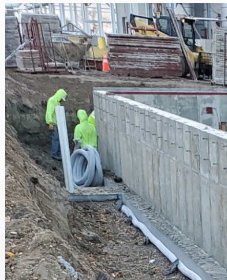
Installing drain tile around the base of the scale before backfilling
