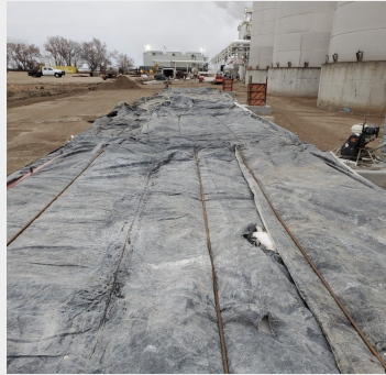
Deck covered with concrete blanket.
